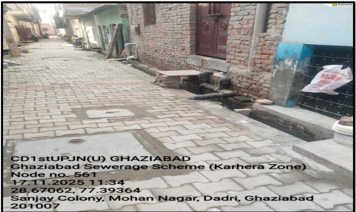
Photograph of sewer laying and road restoration
